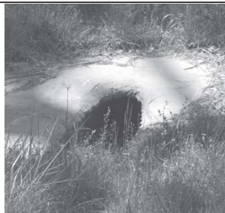
During heavy rains, poorly working culverts can cause flooding that significantly damages roads and bridges. Even during normal wet weather, a crushed or plugged culvert will contribute to the deterioration of the road as it allows water to back up in roadside ditches. Standing water prevents further drainage from the road base and subgrade. A soft base or subgrade will give under
