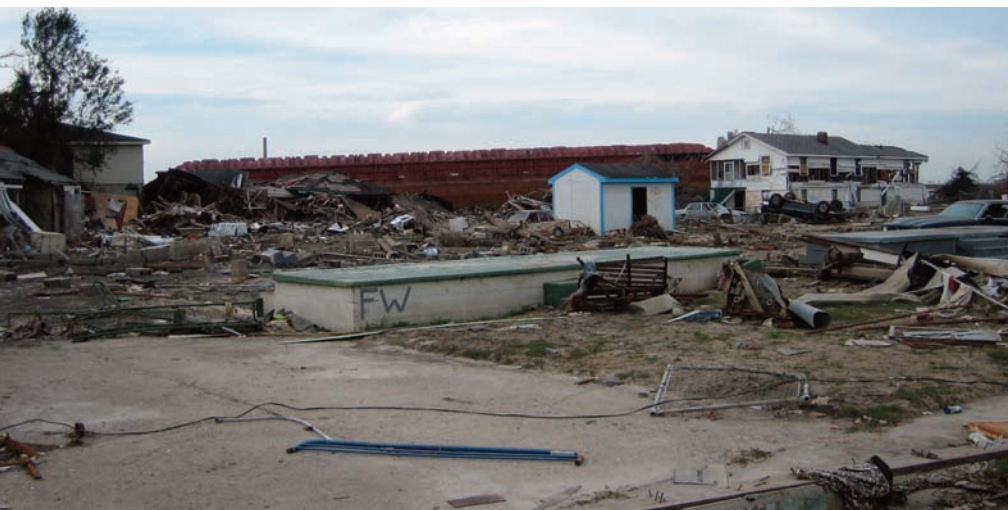
Devastated residential area, Lower 9th Ward, with barge that landed in neighborhood after coming through breach in Industrial Canal visible in background.
